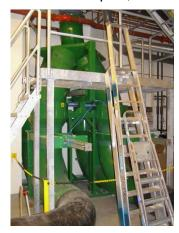
All waste is sorted at source, including at ward level and taken by chute to the basement area; exhaust systems remove odours while waste is awaiting removal.
