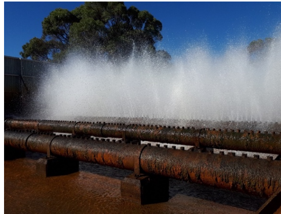
Figure 2.4: Aerosol formation and dispersion from an operational open spray aerator.
