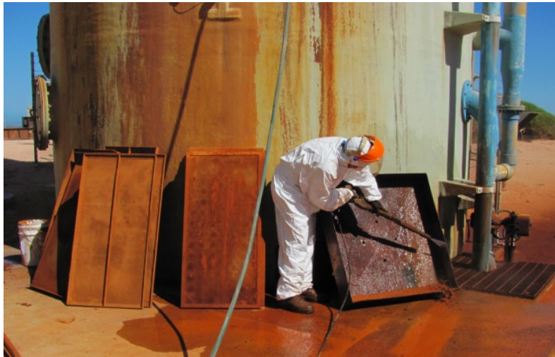
Figure 3.5 – Tray aerator mesh decoupled and cleaned at floor level (photo provided by WCWA)
