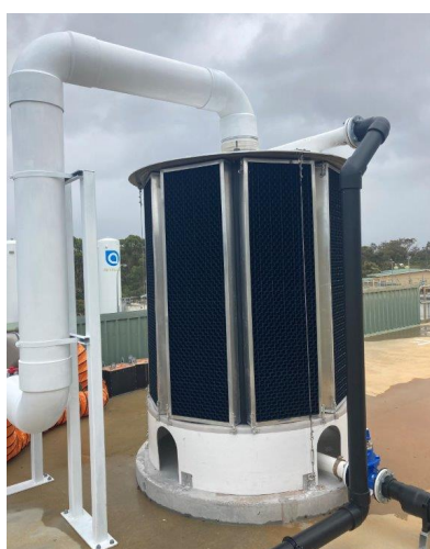
Figure 7.2: Improved aerator design recently tested at GWTPS in Western Australia
