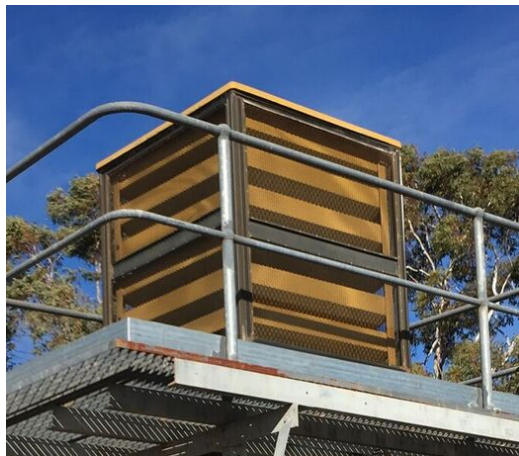
Figure 2.3: Tray aerator operated in groundwater treatment plant
