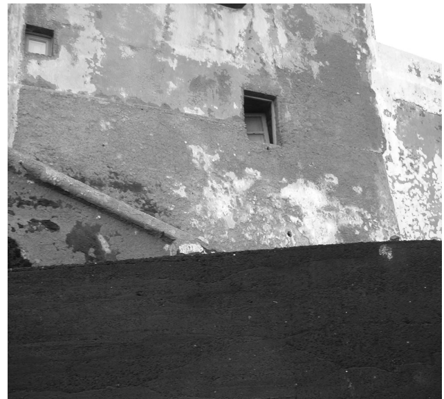
Fig. 8. View from north-west of building #1, at Piscità (Stromboli – Fig. 4). The picture was taken few days after the 2002 tsunami. The only visible damage is an unhinged window on first floor. The PTVA-3 Model classified building #1 as having a “very low” RVI score which correlates well with the actual damage sustained by this building.
