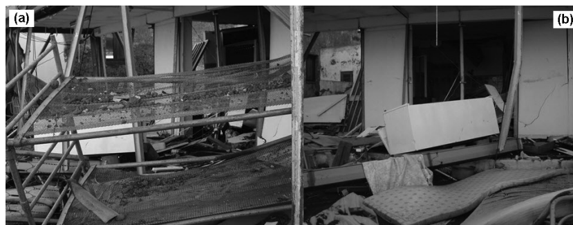
Fig. 12. Two pictures of building #5 (Punta Lena, Stromboli – Fig. 6) taken after the 2002 tsunami. The flow broke doors and windows, penetrated indoors and dragged the building contents outside (a). A large crack can be observed in the front side wall (b). However, that wall does not appear to be part of the load-bearing structure of the building, as does the undamaged column at its right. The PTVA-3 Model classified building #5 as having an “average” RVI score.
