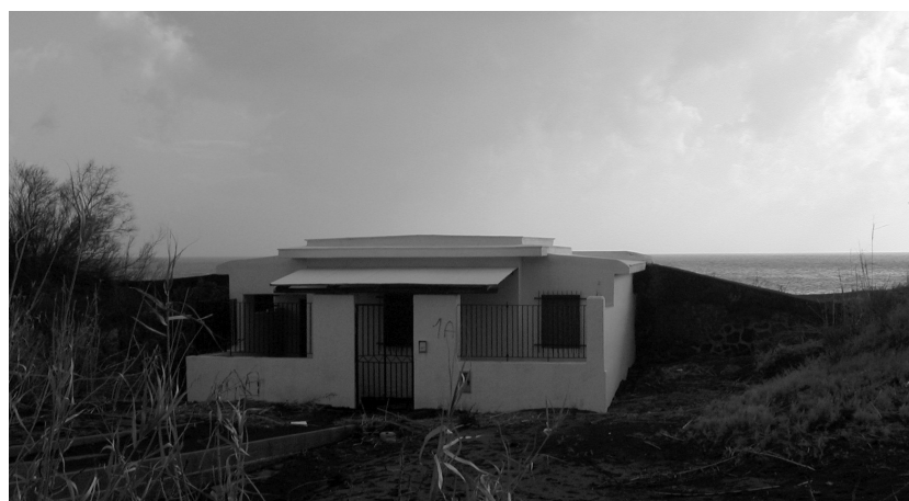
Fig. 13. View of the western side of building #6. The picture was taken a few days after the 2002 tsunami. Building #6 is a Coastguard station on the beach of Scari (Stromboli – Fig. 6). As clearly shown by the picture, the seaward side of the building is totally “covered” by a coastal dune. The PTVA-3 Model attributed to building #6 an “average” RVI score.
