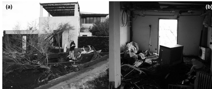
Fig. 9. Pictures of building #2, at the eastern end of Ficogrande (Stromboli – Fig. 5), taken after the 2002 tsunami. (a) A view of the building from north-west. (b) Damage to the interior. The PTVA-3 Model classified building #2 as having an “average” RVI score.
