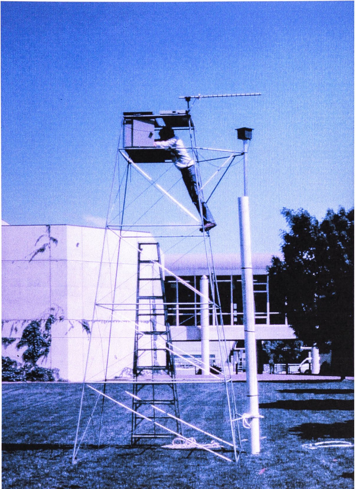
Figure 2.16 Space frame tower shown before installation. About half the space frame would be submerged in the lake.
