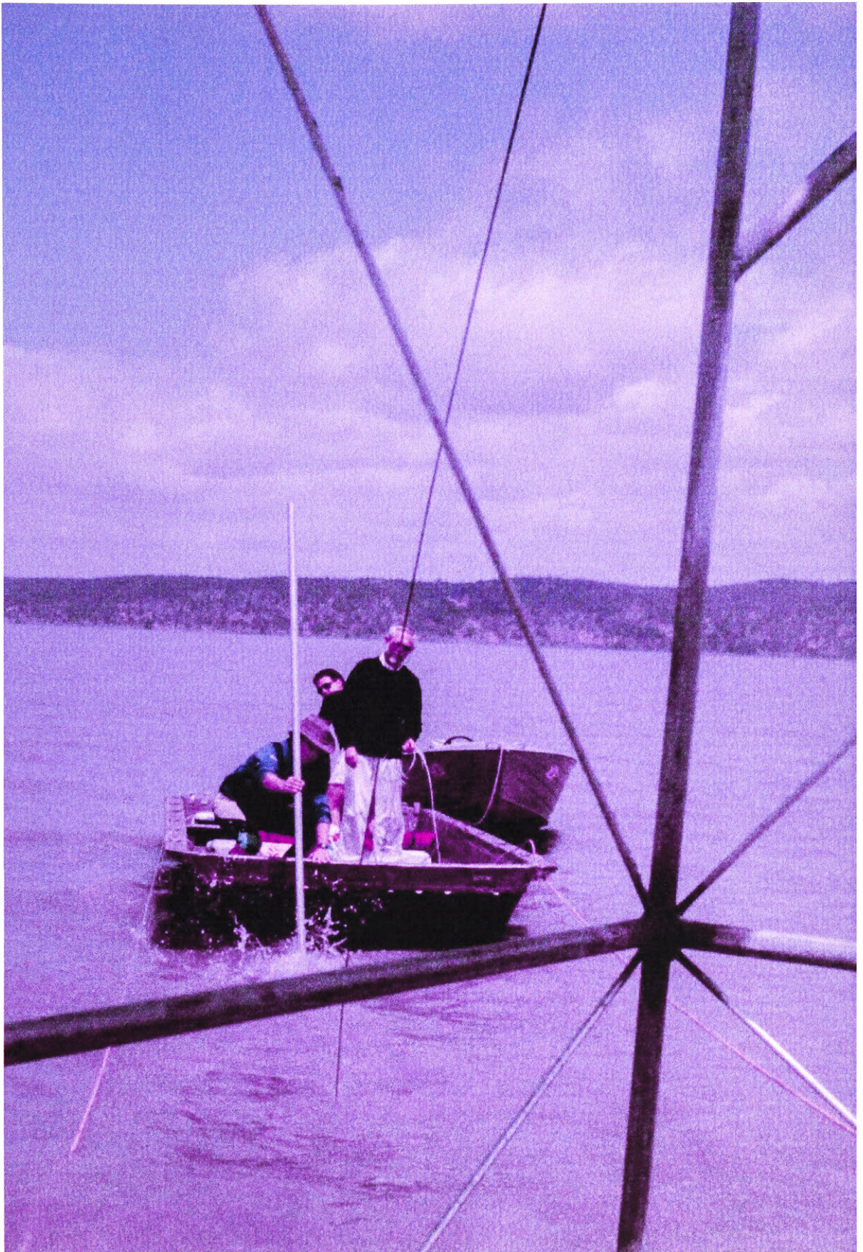
Figure 2.17 Hammering of one of the anchors into the lake bed. Note the guy wire still hanging loose.
