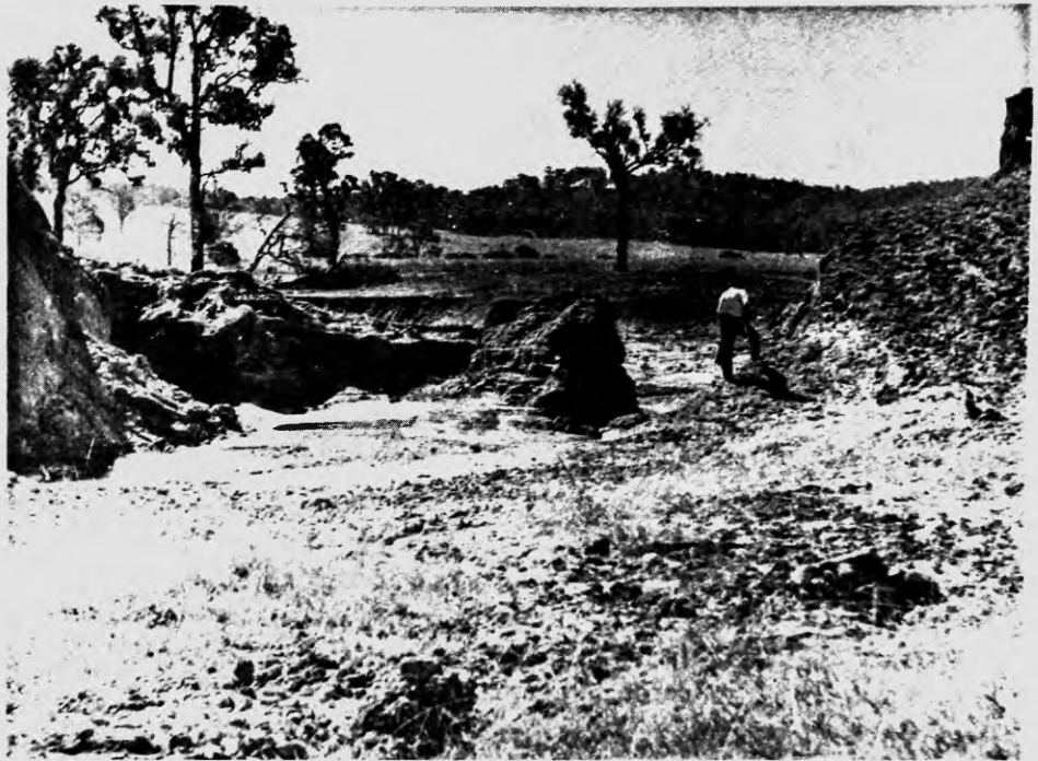
Fig. 1: Dam failure at Liverpool, N.S.W. Cause of failure – inadequate compaction at extremely low moisture content.
