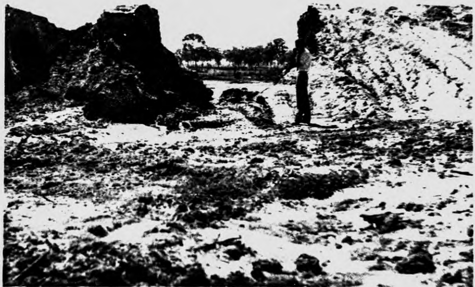
Fig. 2: Dam failure at Bribbaree, N.S.W. Cause of failure – presence of solodic soil in embankment.
