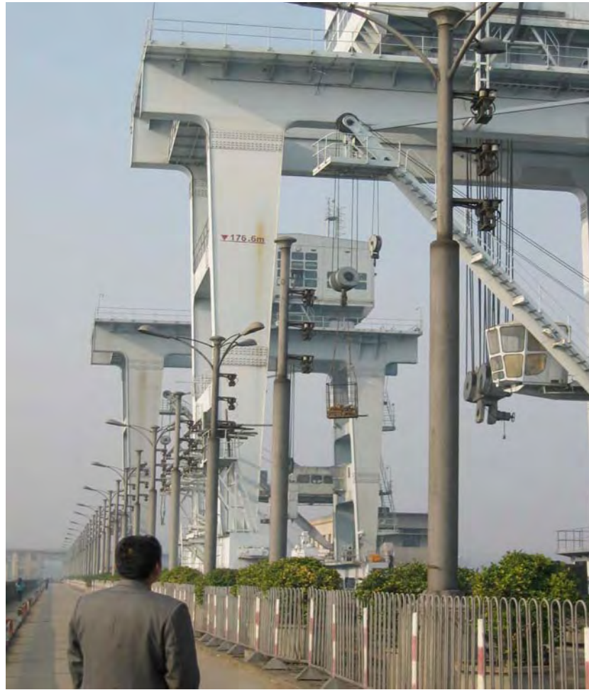
Figure 5.7 Picture of Part of the Superstructure of the Original Danjiangkou Dam (Photograph by author, 2004). (The lettering on the vertical metal girder marks the intended future upper level of the Dam.)
