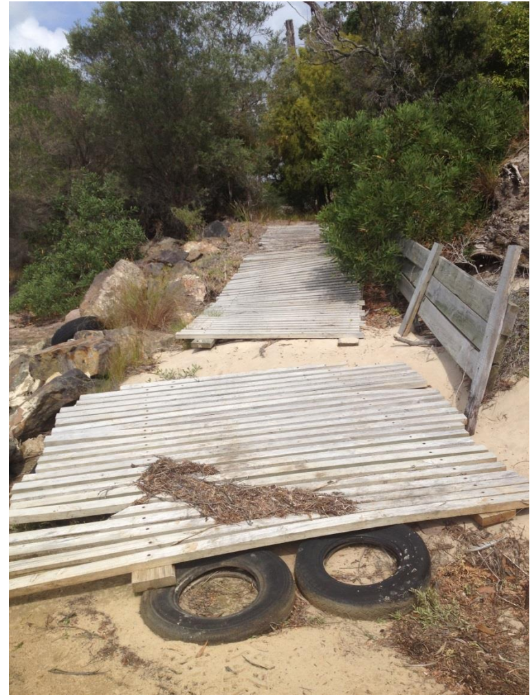
Figure 3.6: Damaged Timber Slatted Boat Ramp
