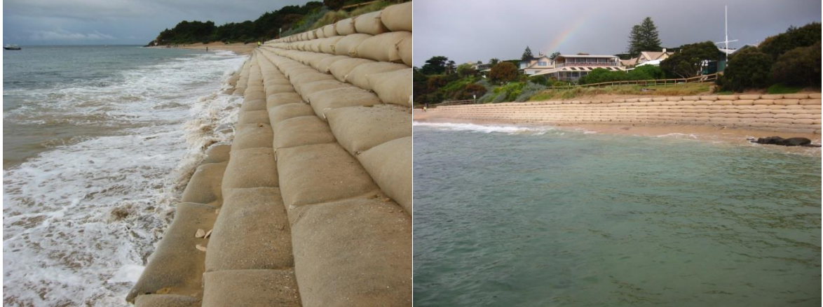
Figure 8.1: Typical Engineered Geotextile Container Revetment, Portsea, Victoria
