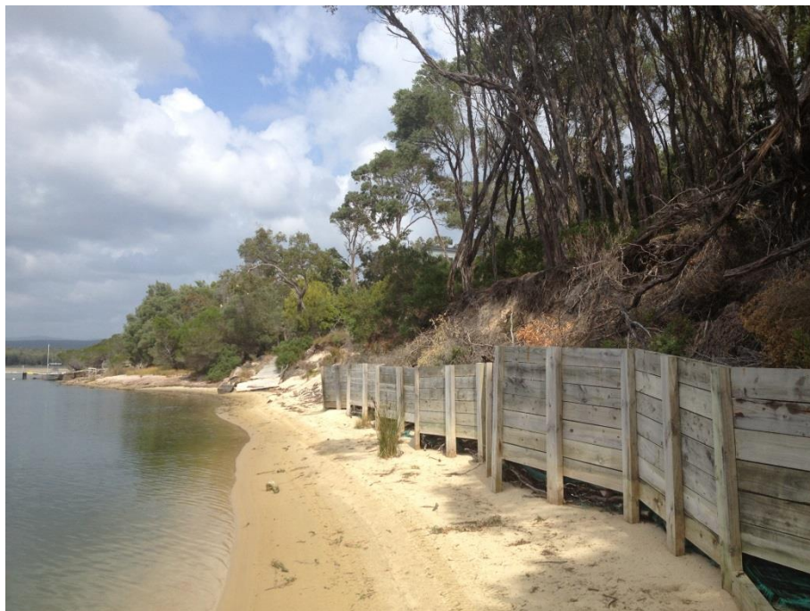
Figure 3.4: Existing Treated Pine Sleeper Seawall (Looking West)
