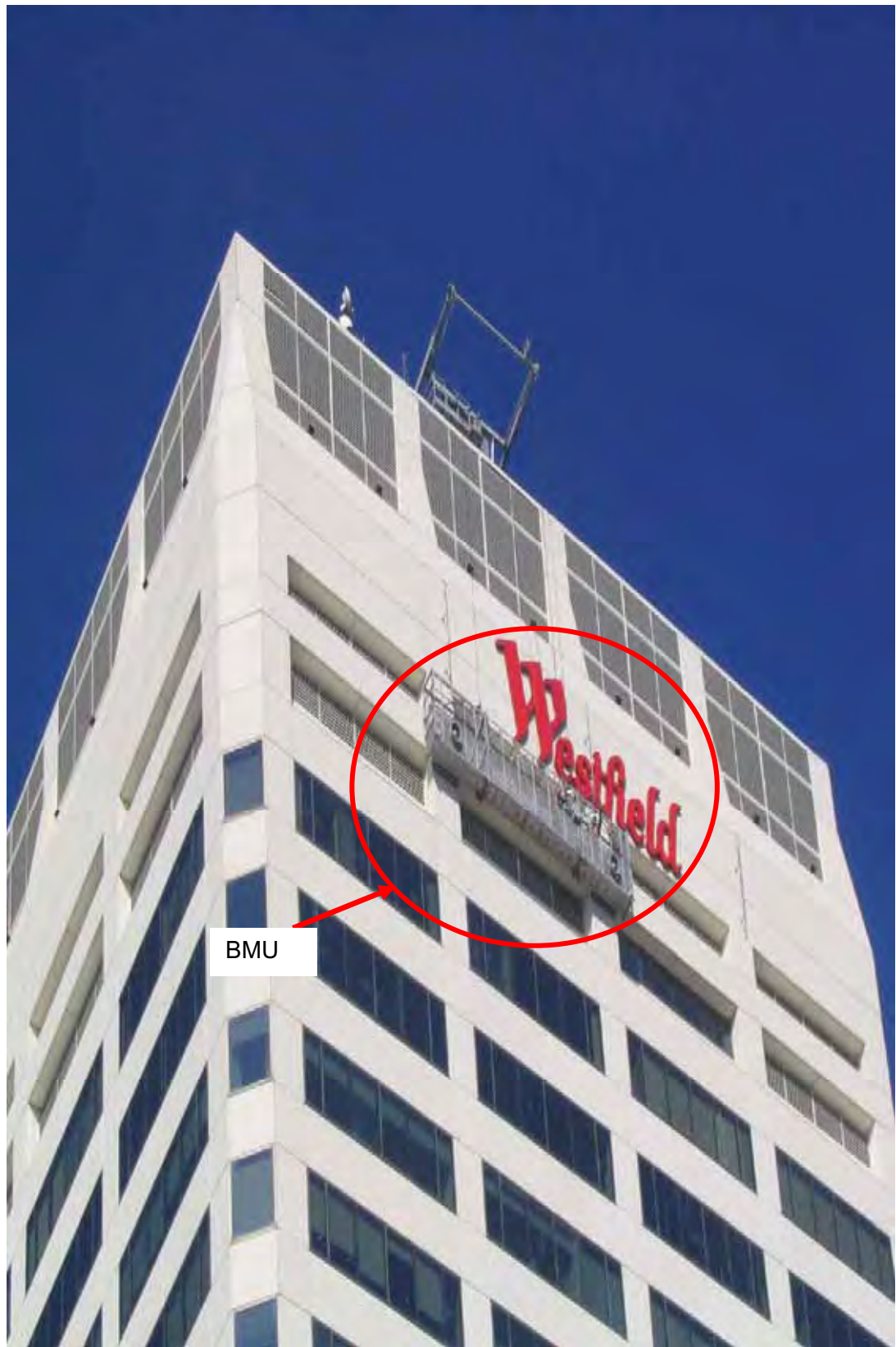
Figure 4.69 BMU situated at level 26 while Perfect Engineering Pty. Ltd. engaged in refurbishment.
