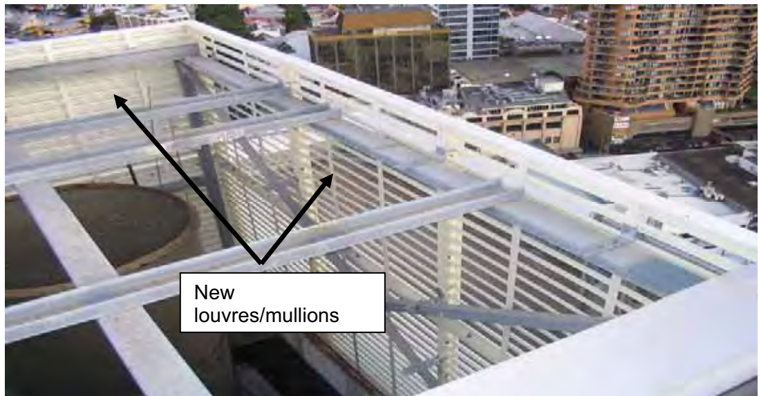
Figure 4.49b Top view of new southwest louvre section, showing details of connections installed at every major structural position.
