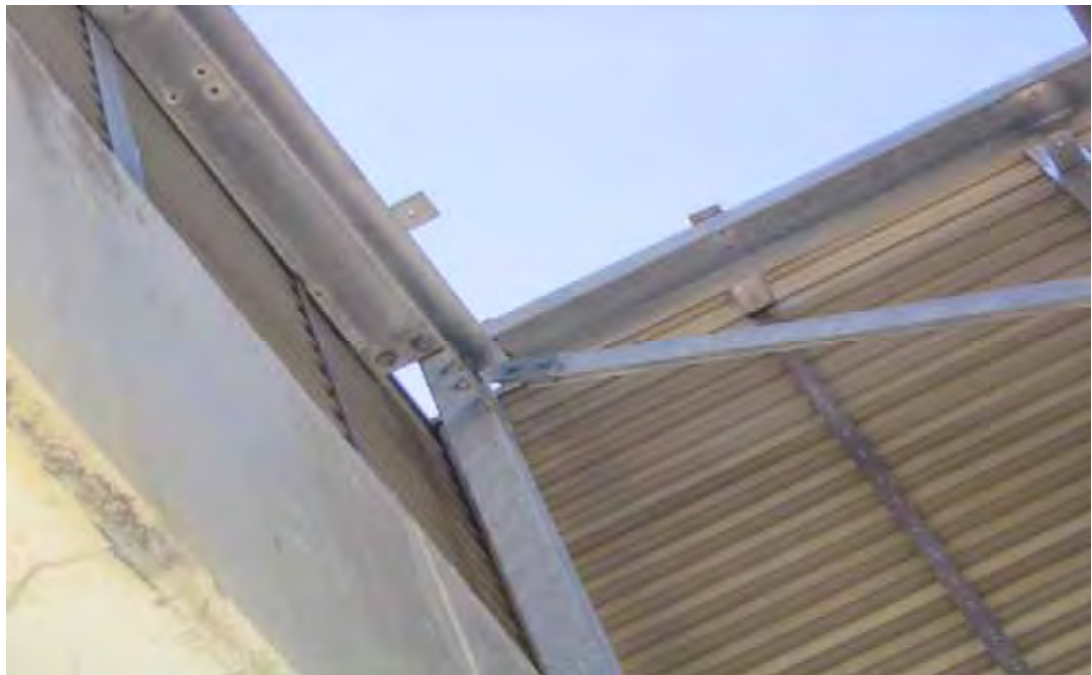
Figure 4.26 Corroded bolts replaced with new structural galvanised bolts; old brackets held onto PFC using one or two corroded bolts; brackets held to structural mullion with one or two tek screws.
