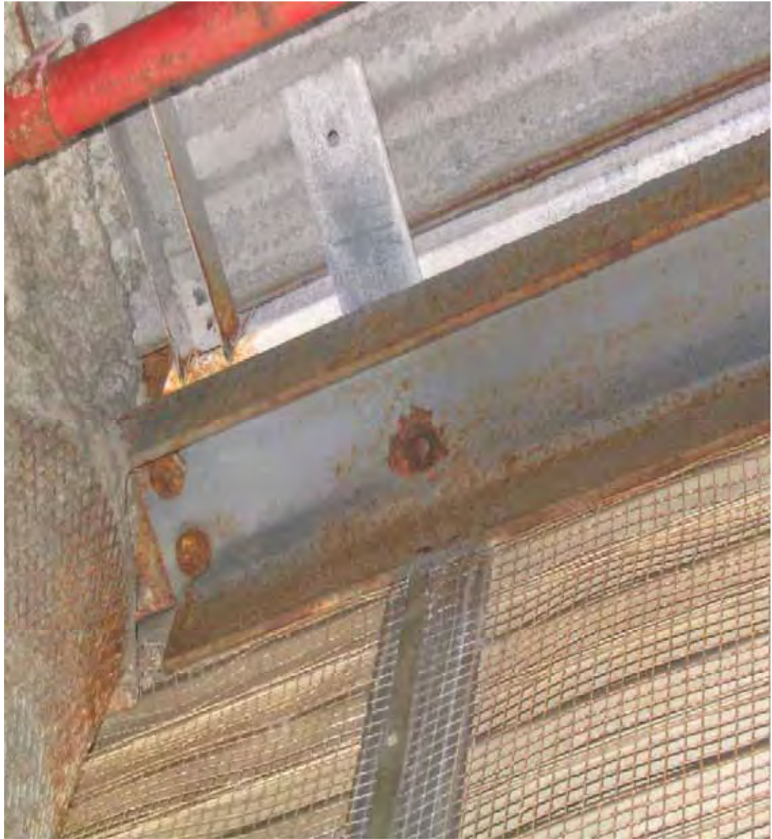
Figure 4.23 Corroded bolts and corroded PFCs as main structural supports for louvres on level 29; roof and horizontal PFC encourage indefinite corrosion deposits.
