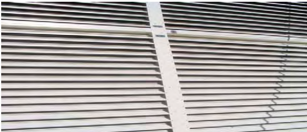
Figure 4.62 Two mullion sections and louvres connected and held securely in place on level 28.
