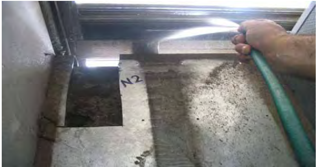
Figure 4.19 Preparation and cleaning of mullions adjacent to baffles.
