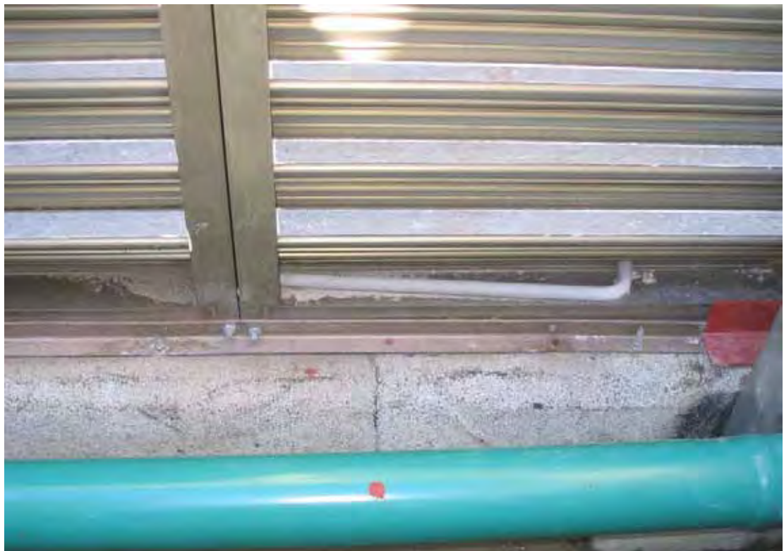
Figure 4.38b M8 galvanised bolts connecting to existing equal angle with M8 chemically set bolts into equal angle and hob for extra strength against wind uplift or lateral forces.
