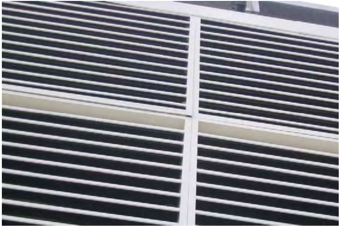
Figure 4.33 One of four typical louvre panels sitting loose due to incorrect and inadequate connection.
