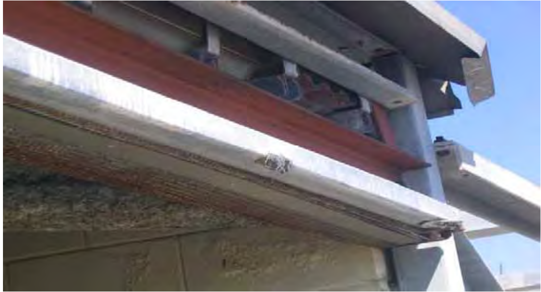
Figure 4.25a Structural beam holding roof with inadequate support beneath should existing corrosion continue at same rate.
