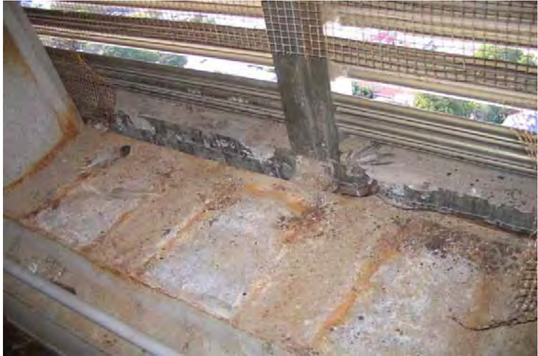
Figure 4.17 Steel cladding extending from base of baffles and enveloping face mullion, causing galvanic corrosion.
