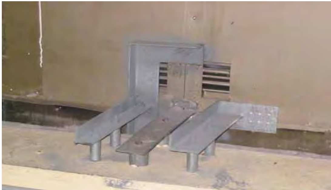
Figure 4.21 Typical C-brackets, left-hand side fabricated and hot dip galvanised for lower sections of level 28; additional brackets on right-hand side wall support remainder of mullions.
