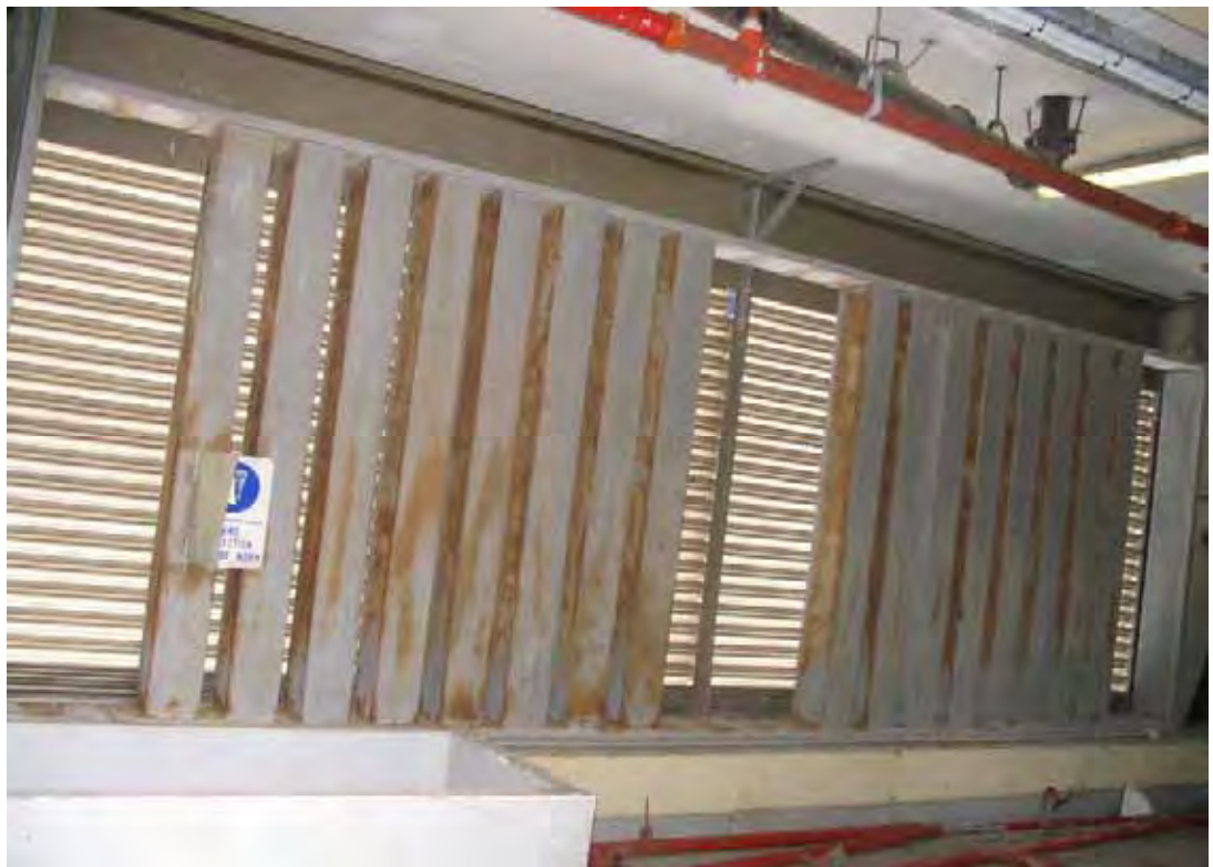
Figure 4.16 Corroded noise attenuators or baffles adjacent to louvers on north, south, and southeast sections of level 28.
