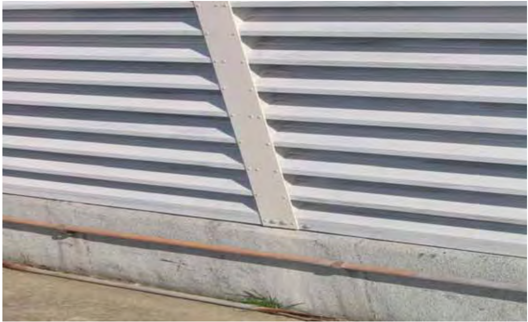
Figure 4.38a M8 bolts connecting to equal angle on hob on other side.
