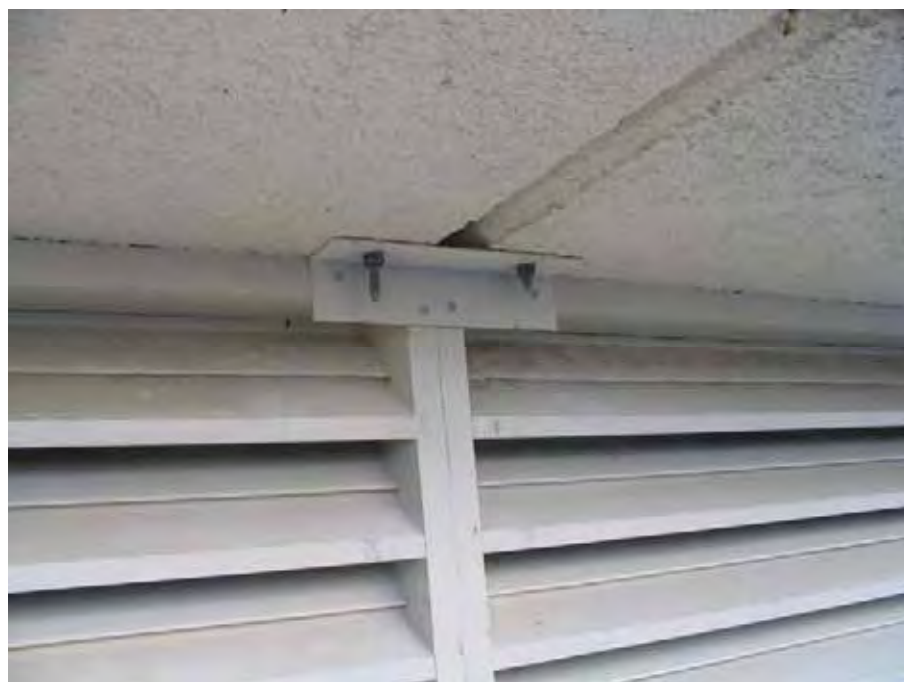
Figure 4.67 Aluminium equal angle 60 mm x 60 mm x 3 mm 6060 T5 chemically anchored to concrete roof to hold louvre mullion sections in centre.
