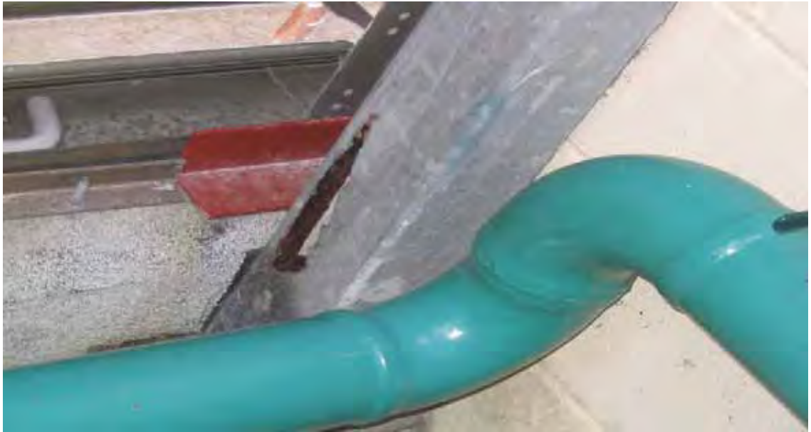
Figure 4.39 Corroded column on southern face near western section owing to holes' not being plugged on top of columns after galvanising during original fabrication.
