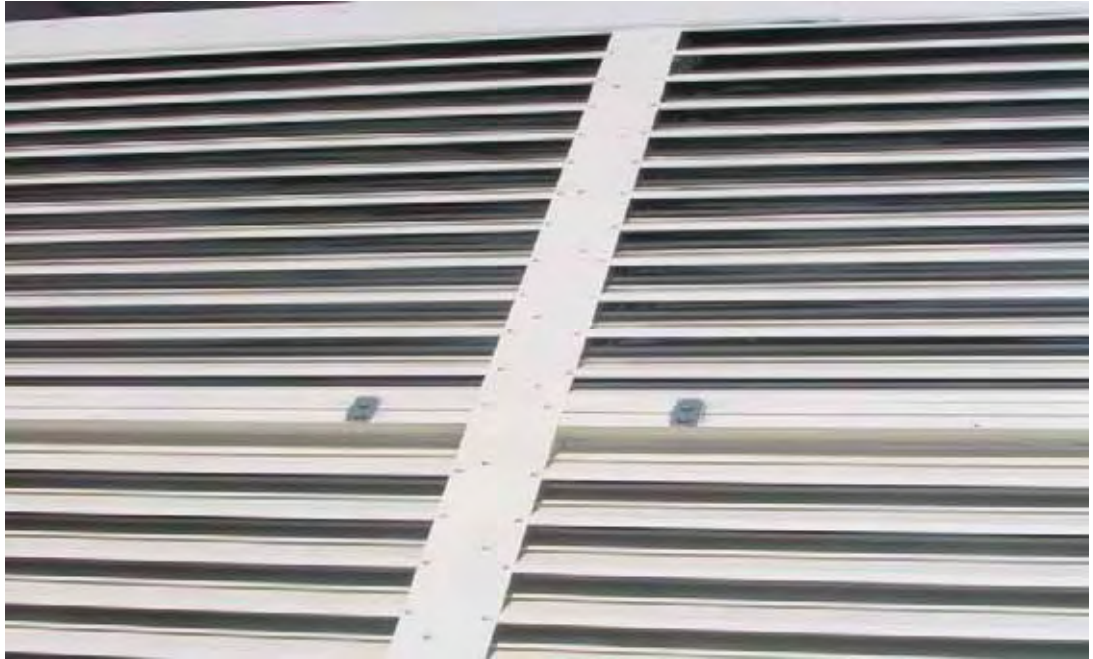
Figure 4.58 Parapet cladding sitting over mullion face of louvres, providing additional connection for louvres; holes drilled in horizontal portion of mullions to allow entrapped water to escape.
