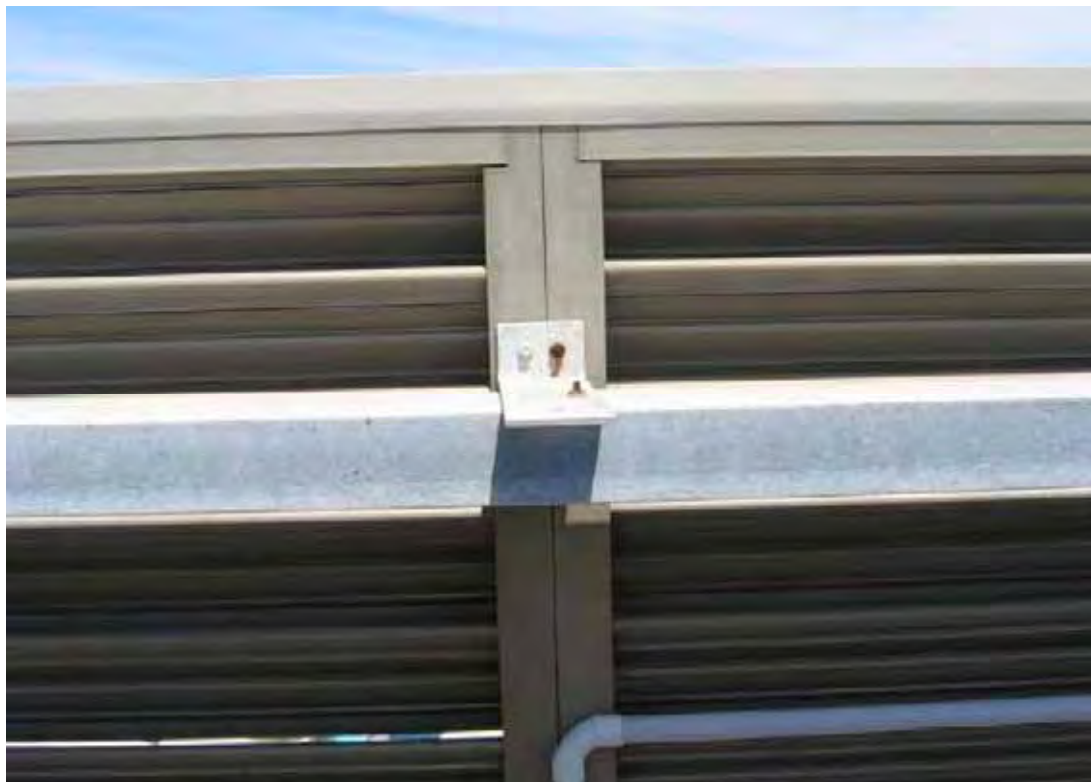
Figure 4.28 Corroded 6 mm tek screws barely holding structural louvres through rounded brackets; typically one corroded bolt connected to the structural PFC; one of principal reasons for failure of southwest corner.
