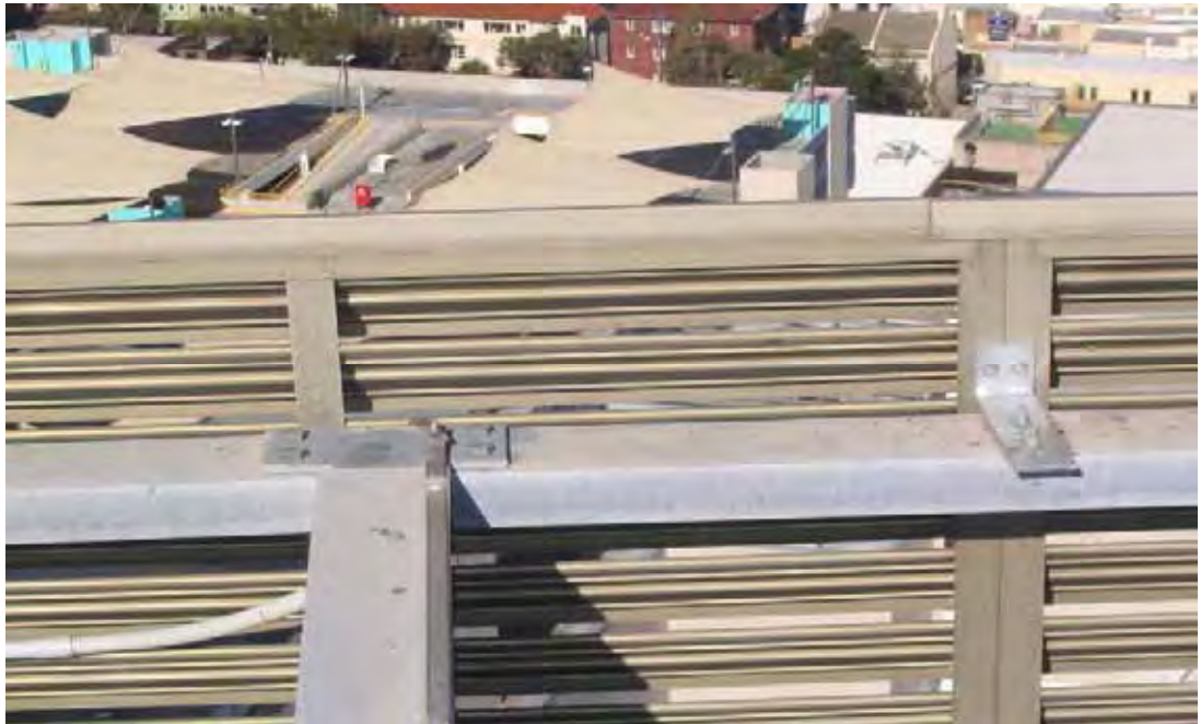
Figure 4.41 Holes on column left hand side plugged with special two-mix steel putty.
