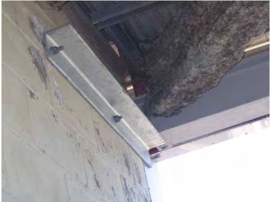
Figure 4.25c Hot dipped galvanised structural angle chemset into wall directly beneath beam for additional support.
