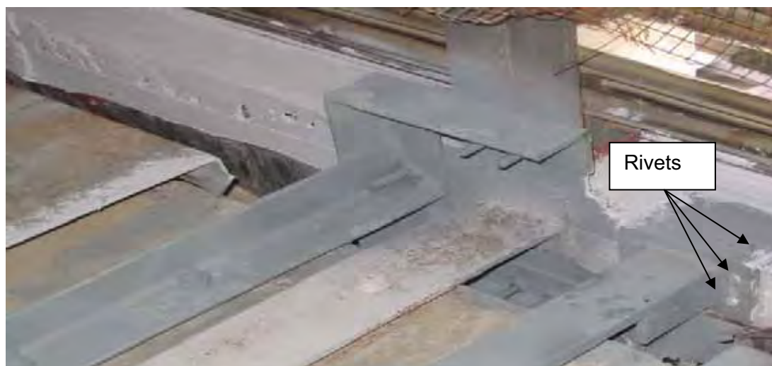
Figure 4.64b Lower C-bracket connecting mullion in internal of level 28 using six bolts; jigs placed on outside for abseilers to drill through mullions and bolt directly through welded nut sitting on face of brackets.
