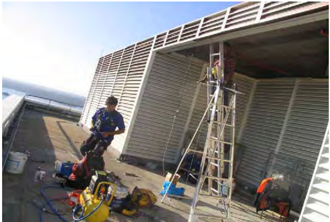
Figure 4.54 New louvre panels fabricated to replace old damaged louvre panels in BMU garage.
