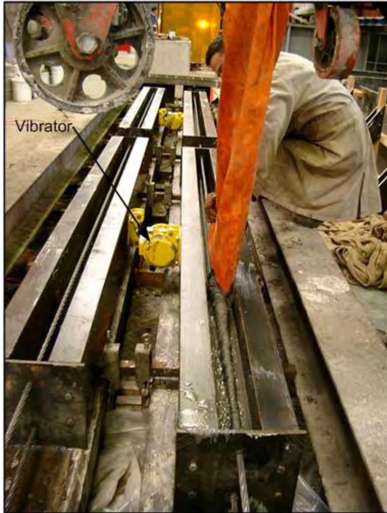
**Figure 3.6:** Prestressed beam construction
