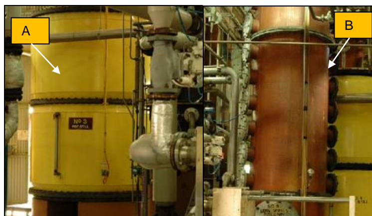
Figure 2.3 Distillation at The Bundaberg Distilling Company, Bundaberg, Australia. (a) Pot still, (b) column still. (Photo D. Flett)
