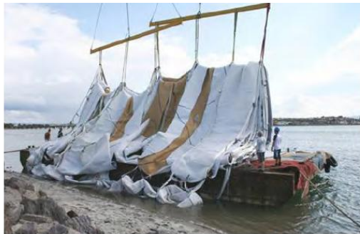
Loading Reef Panel onto Barge
