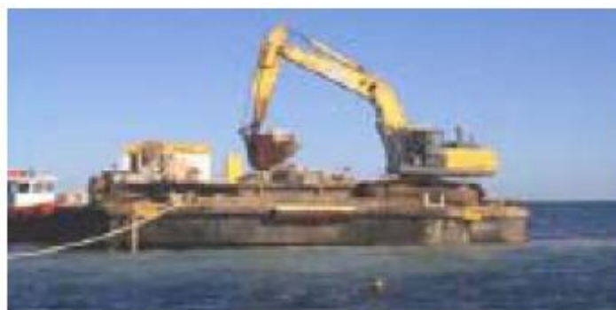
Figure 2.14: Placing Rock on the Cable Station Reef by Barge Mounted Excavator (Jackson and Corbett, 2007)
