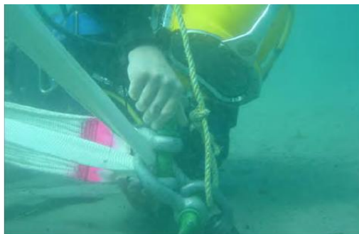
Securing Reef Panel to Seabed Anchor
