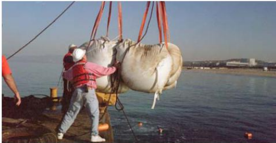
Figure 2.19: Placement of Smaller Geotextile Bags by Sling at Pratte's Reef (Borrero and Nelson, 2003; Jackson and Corbett, 2007)
