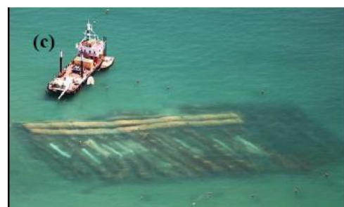
Figure 2.17: Construction of the Boscombe MPR (Mead et al. , 2010)
