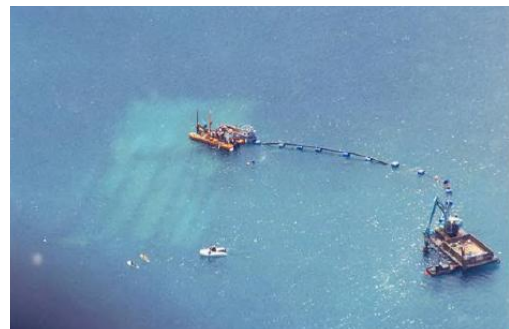
Filling Geotextile Tubes
