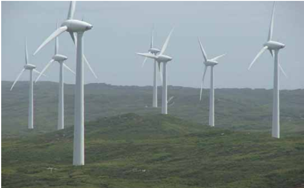
Figure 2.4: The Albany wind farm in Western Australia, Australia. Its turbines have a rated capacity of 1.8 MW with 65-m tower and three 35-m long blades (Verve Energy, 2006).
