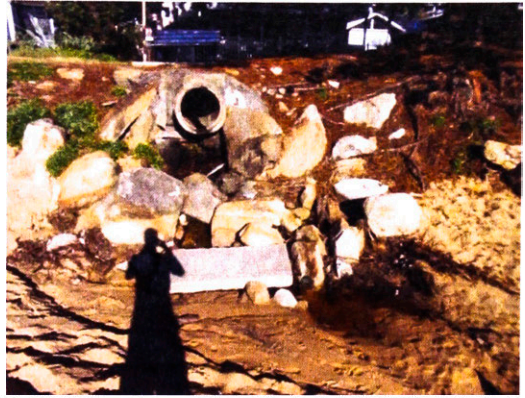
j) Stormwater outlet and scour protection in the centre of the beach
