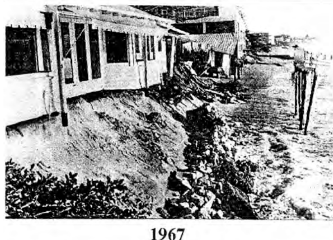
Figure 12. Present condition of the nonengineered revetment that is in place to protect beachfront property at the site of the newly installed ARGUS station at Narrabeen Beach, NSW (Source: Warringah Council).
