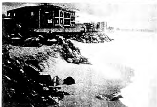
Figure 12. Present condition of the nonengineered revetment that is in place to protect beachfront property at the site of the newly installed ARGUS station at Narrabeen Beach, NSW (Source: Warringah Council).
