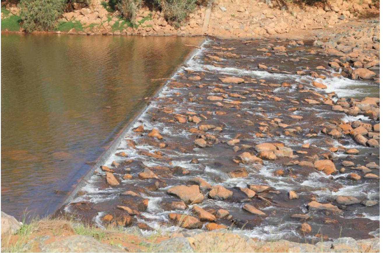
Figure 4.16 Recharge weir constructed across the Ashburton River at Minderoo, Western Australia (Koenigluck, 2015).
