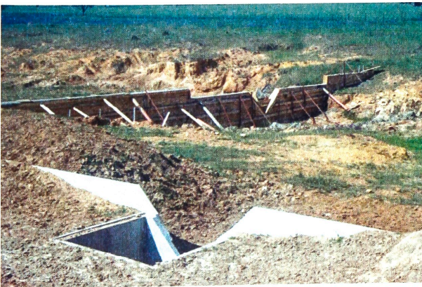
Figure 1.4: Construction of the main weir and a subsidiary weir on a contributing channel
