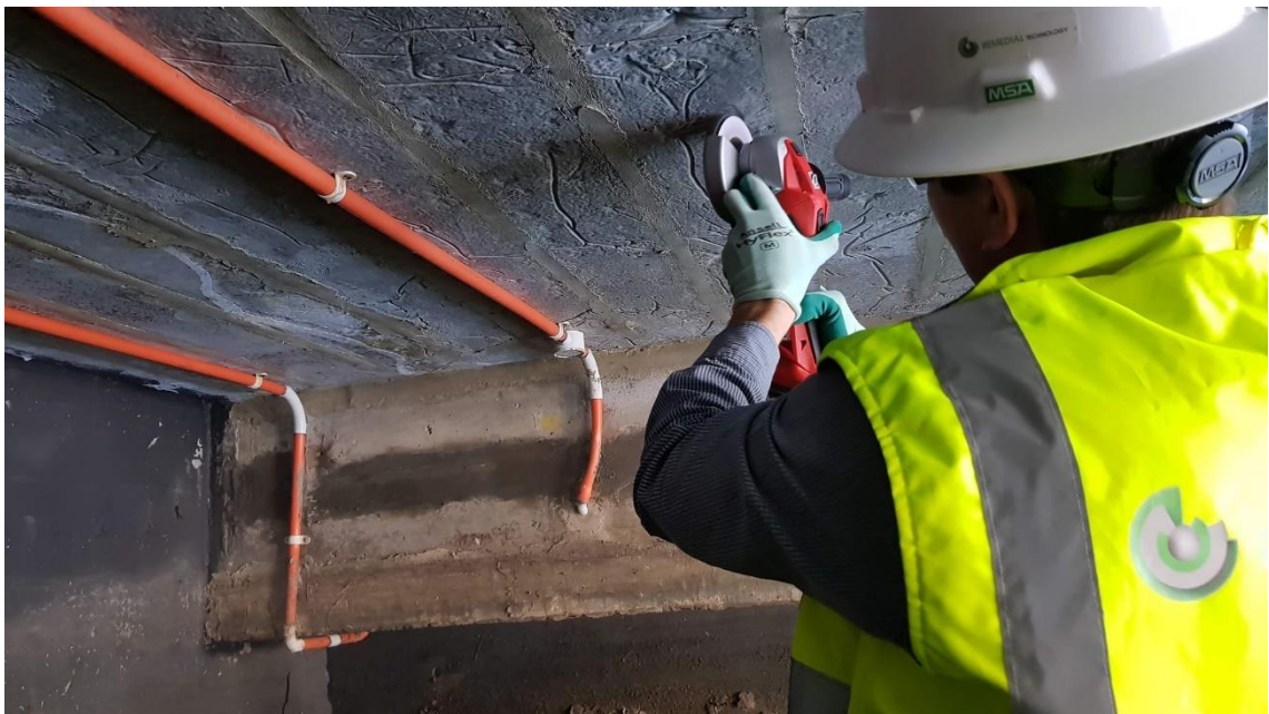
Figure 5.5 – Cleaning of surface using angle grinder
