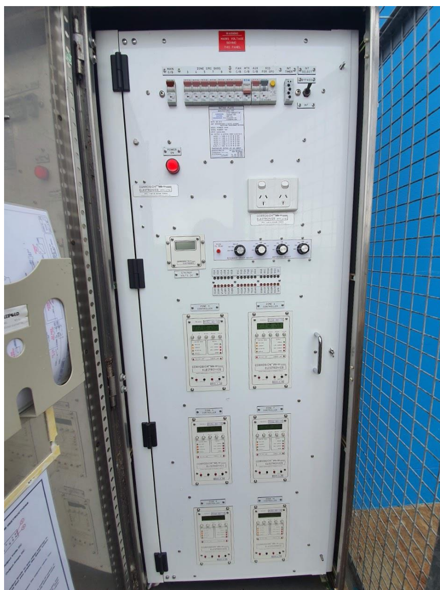
Figure 5.2 - Photo of cathodic protection transformer rectifier unit
