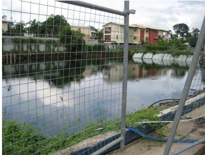
Figure 5.6: The ‘bath tub’ site, Palmer Street, an example of premature site priming with the excavation of a car park below water table that then sat idle (Drane 2014)
